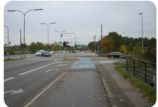
At this unsignalized right turn, the cycle track has dropped to a bike lane with blue coloration and pavement markings through the conflict area.
